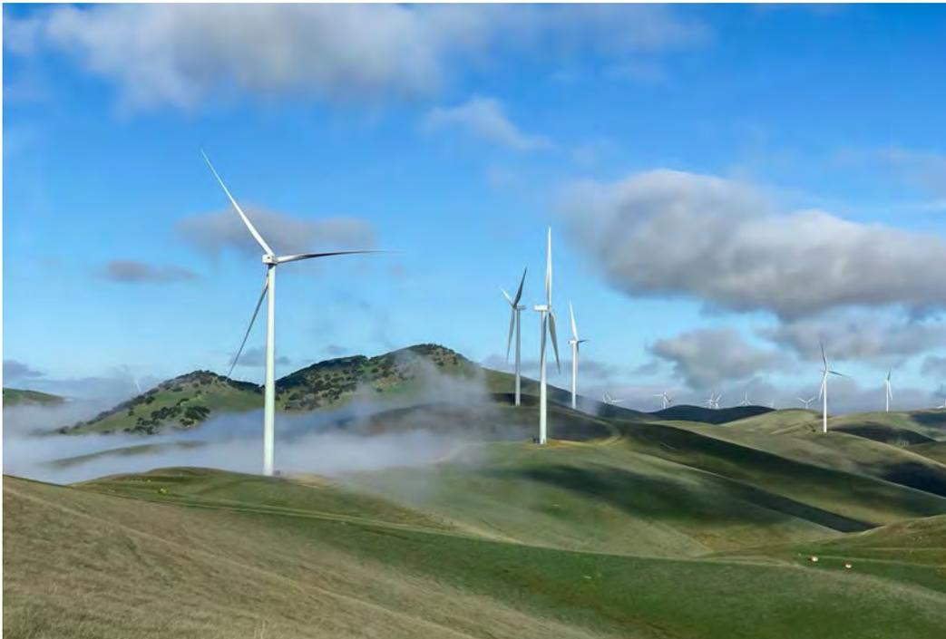
The 57.5 MW Scott Haggerty Wind Energy Center near Livermore, in East Bay Community Energy's service area. The project, named after EBCE's former board chair, is set to go live in the second quarter of 2021. It replaces 569, 100 Kw turbines with 23, 2.5 MW turbines. Photo credit: Salka Energy
